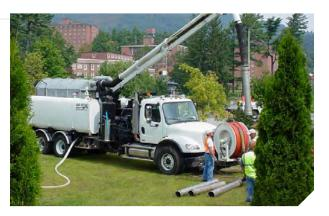
After it reaches a predetermined distance or "step" it is pulled back to the downstream manhole by the hose reel. The debris is removed from the manhole by a downhole submersible pump.
